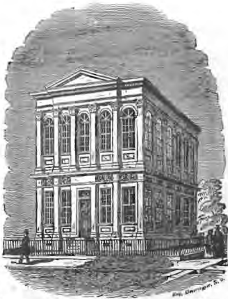
FIG. 11. NEW ORLEANS SCHOOL OF MEDICINE, CORNER OF TULANE AVENUE AND VILLERE STREET, OPPOSITE THE CHARITY HOSPITAL.
